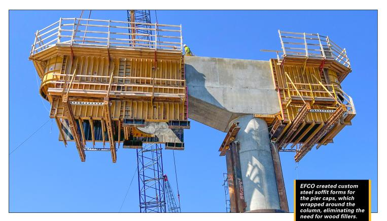
safely on the ground and flying them into place with fewer crane picks, increasing jobsite productivity. The formwork for each pier cap was lifted in one crane pick. Once the concrete was placed for the pier caps, the formwork was stripped in two crane picks, with each gang being lowered to the temporary bridge.
