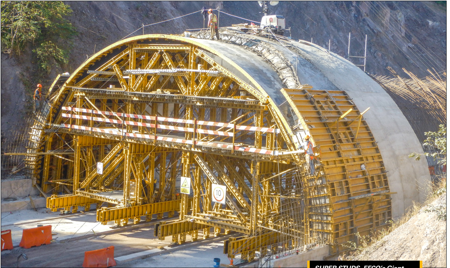
SUPER STUDS, EFCO's Giant Steel Erector Set, configure easily into a support frame for the REDI-RADIUS forms.
