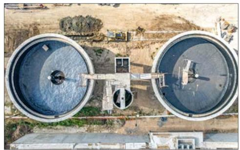
The completed plant will process between 10,463 to 15,695 yd3 (8,000 and 12,000 m3) of industrial liquids per day for the tanneries in the industrial park.
