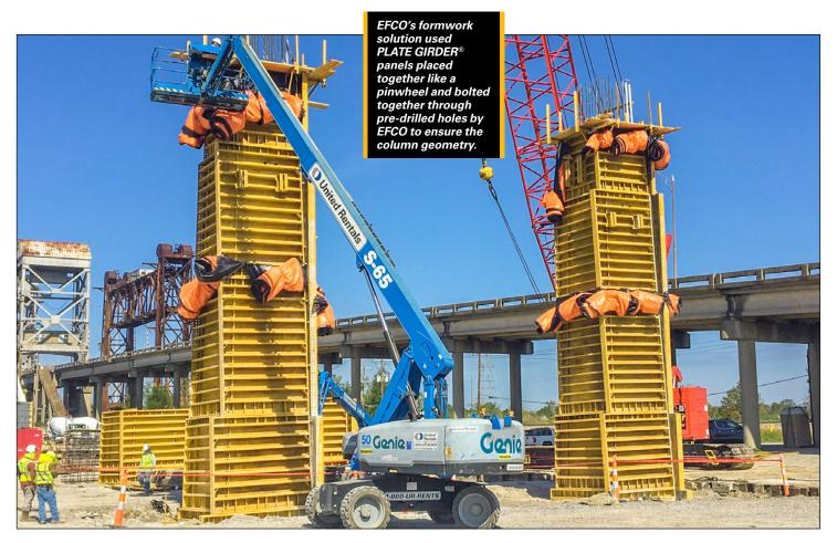
A pour bridge made from EFCO <u>SUPER</u> <u>STUDS</u><sup>®</sup> and <u>E-BEAMS</u><sup>®</sup> was custom-built for the crew to have access between the two columns during the dual-column pour.
